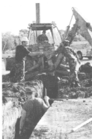
Members work to make ready one of the trenches to house wiring for the campus' electric infrastructure.
