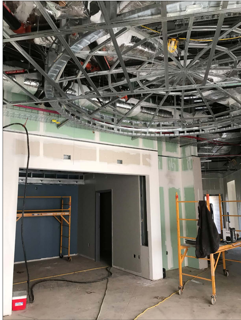
The main entry area, with the SARM desk yet to be installed in the opening at the bottom left.
