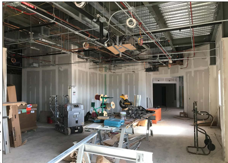
The main 970th command section area, which will be filled with semi-permanent walls later on in construction.
