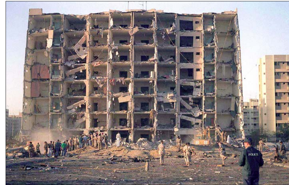
Nineteen Airmen died and more than 350 were injured in the terrorist attack at Khobar Towers in Dhahran, Saudi Arabia, on June 25, 1996. The front of Bldg. 131 was blown off when terrorists detonated a fuel truck parked nearby. (Courtesy photo)
